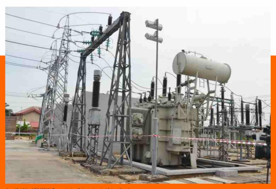
$1 \times 60$  MVA, 132/33KV Transmission Sub-station in Afaha Ube, Itu
